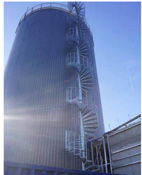
Large-scale storage systems compensate fluctuating network feed-in, Photo: AEE INTEC
