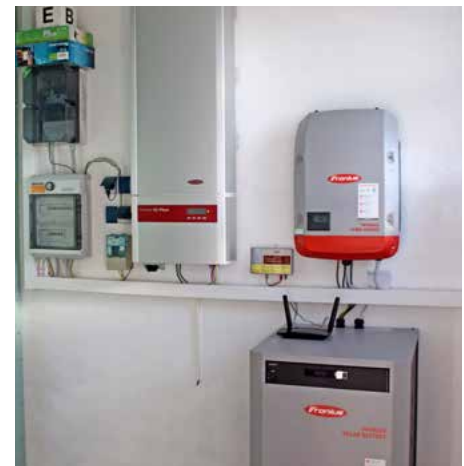
Energy monitor Eberstalzell (left) and residential PV storage system (right), Chart and Photo: Netz Oberösterreich GmbH
