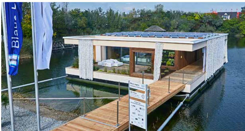
LISI, the plus-energy world champion house, was declared the best solar house in the world at the 2013 Solar Decathlon, an international competition in California. The building was developed and constructed as part of an interdisciplinary project at the TU Wien (Vienna University of Technology), under the direction of Karin Stieldorf from the Faculty of Architecture and Planning. www.solardecathlon.at , Photo: Blaue Lagune/Thomas M. Laimgruber, blauelagune.at
