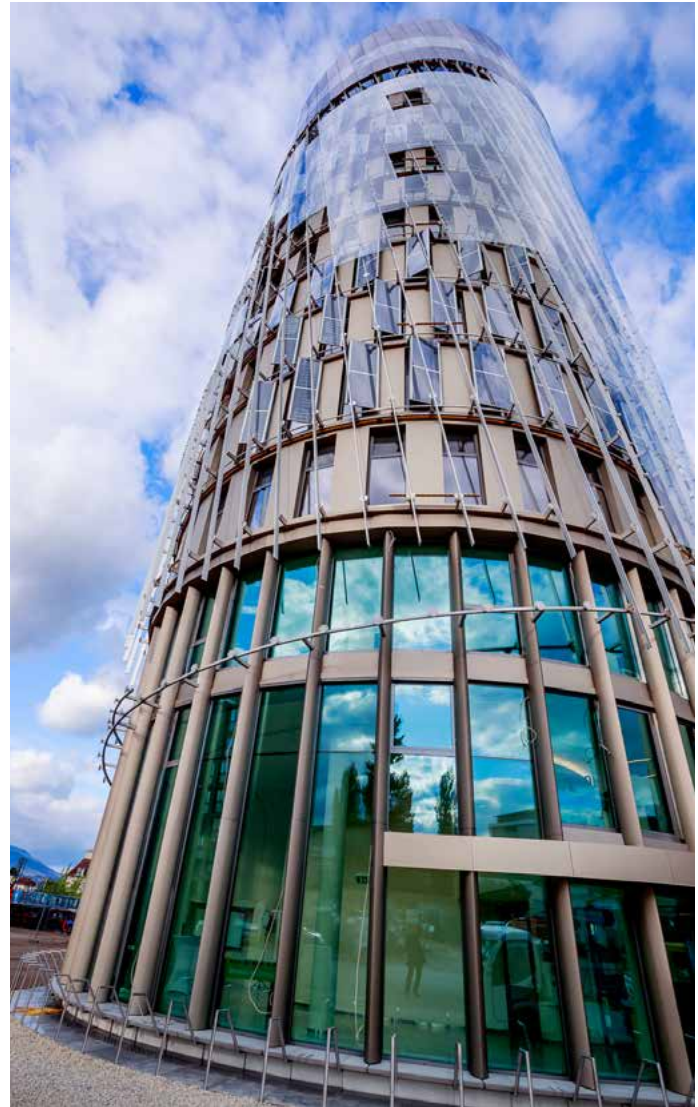
Science Tower – Smart City Graz, Photo: Climate and Energy Fund/Gerhard Buchacher
